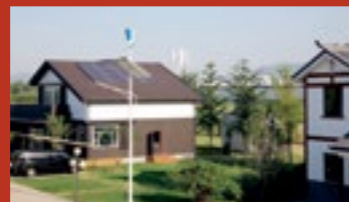
The roof and car shed are equipped with PV modules (total power: 7.54 kW; daily mean generated energy: 24 kWh).
